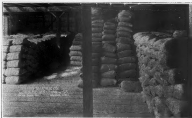
Interior View of the Storage Unit
